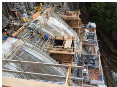
Construction of New Piers 4 and 5
