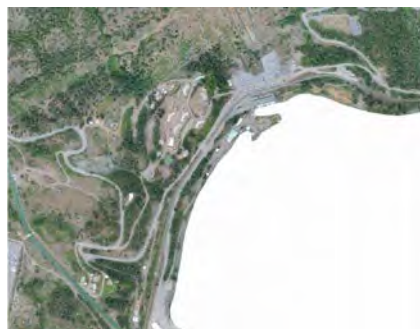
Aerial view of the Bridge powerhouses and penstock slopes
