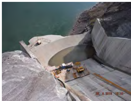
WAC Bennett Dam Spillway Chute - Working Platform Construction
