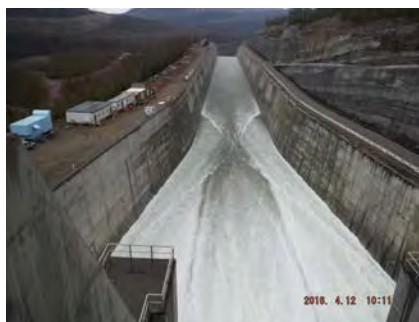
WAC Bennett Dam Spillway Chute- Ice Flushing
