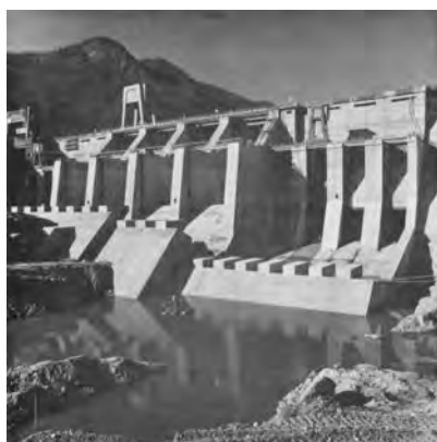
Hugh Keenleyside Low-Level Outlets (right side of photo)
