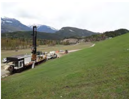
Sonic rig drilling standpipe piezometer
