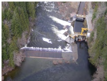
Salmon River Diversion Dam
