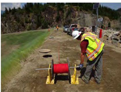
Pulling instrumentation cable
