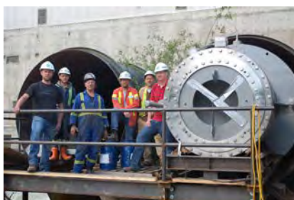
Pressure relief valve upgrade
