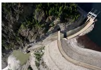
Terzaghi Dam- Spillway and low level outlet tunnel
