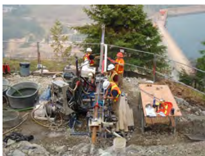
Left Bank Slopes-Instrumentation Installation
