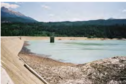
Upstream Shotcrete Face of La Joie Dam
