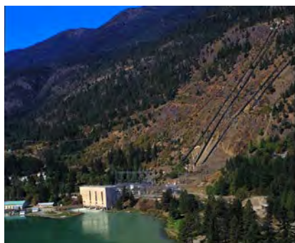
Bridge River 1 - Penstocks
