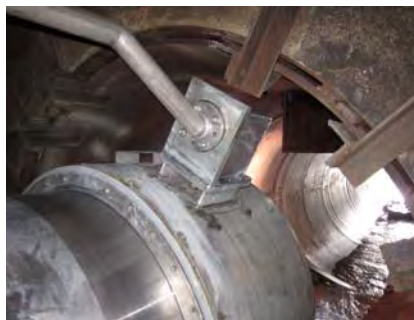
North Conduit drain improvements
