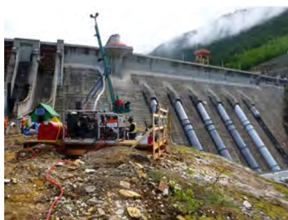
Drilling in the Marble Shear Block
