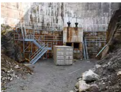
Wilsey Dam-Access and Safety Improvement
