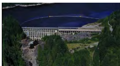
Jordan River Diversion Dam
