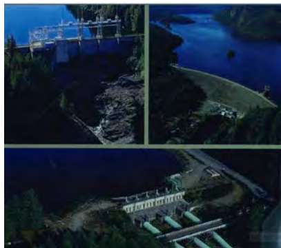
Campbell River System - Dams
