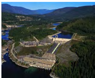
Kootenay Canal Dam and Powerhouse
