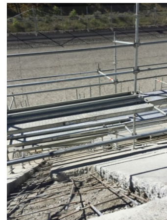
2017 Canal lining repairs
