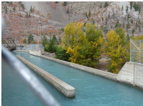
Cayoosh Creek Aqueduct
