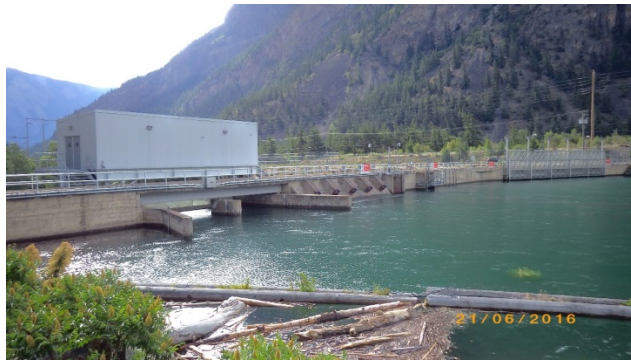
View of Seton Dam from the earthfill dyke
