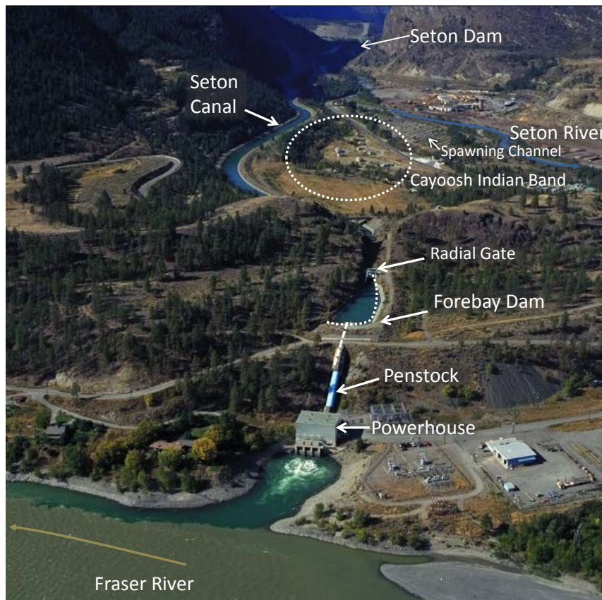
Seton Canal to Powerhouse
