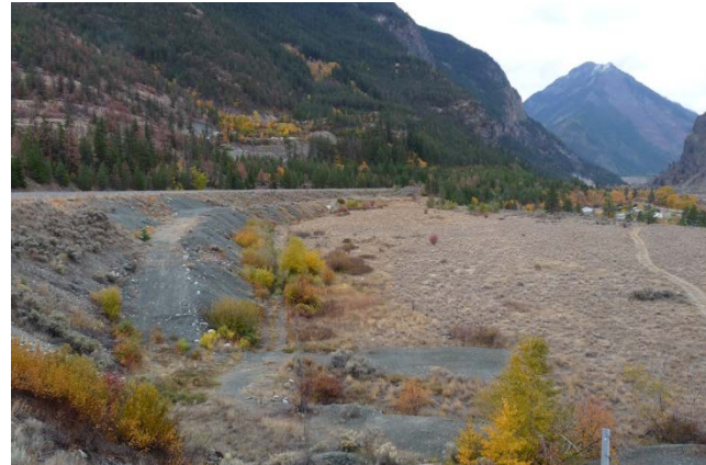
View of Seton Canal embankment adjacent to Cayoosh Band
