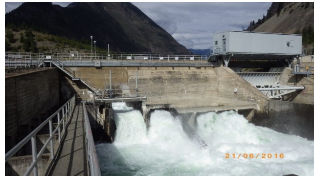
Seton Dam fishwater release gate and siphons in operation
