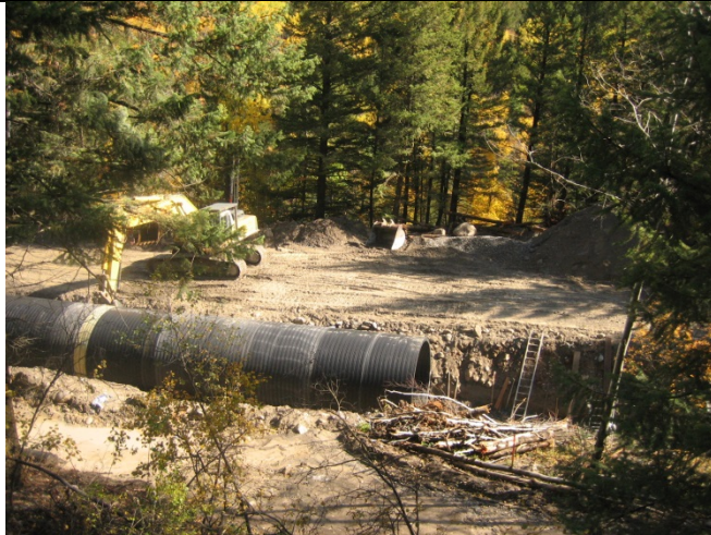
Construction of the new penstock
