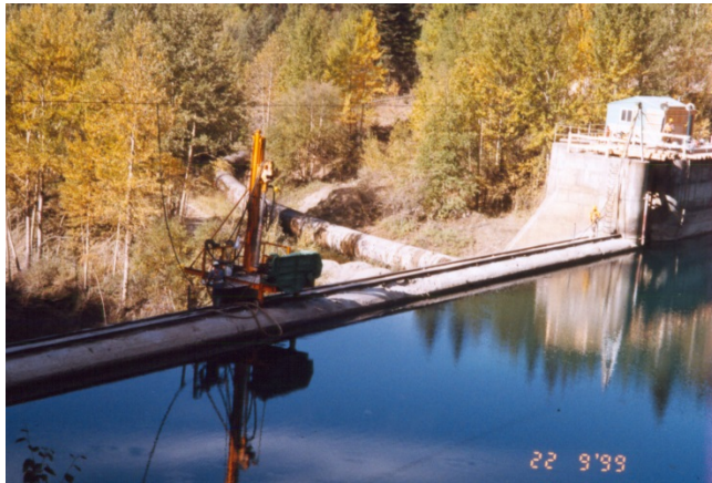
Drilling holes for the post-tensioned anchors
