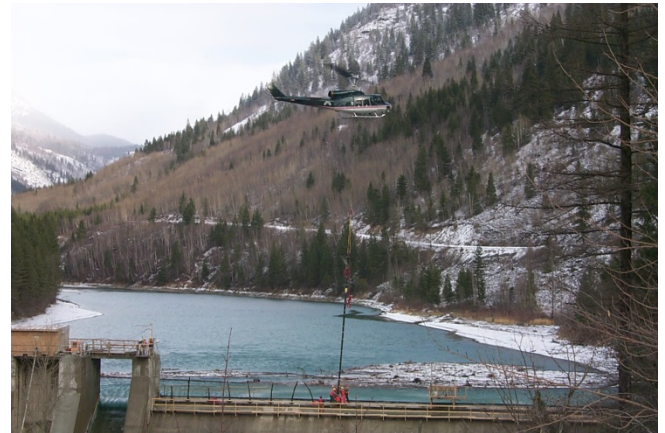
Installation of a post-tensioned anchor in the spillway
