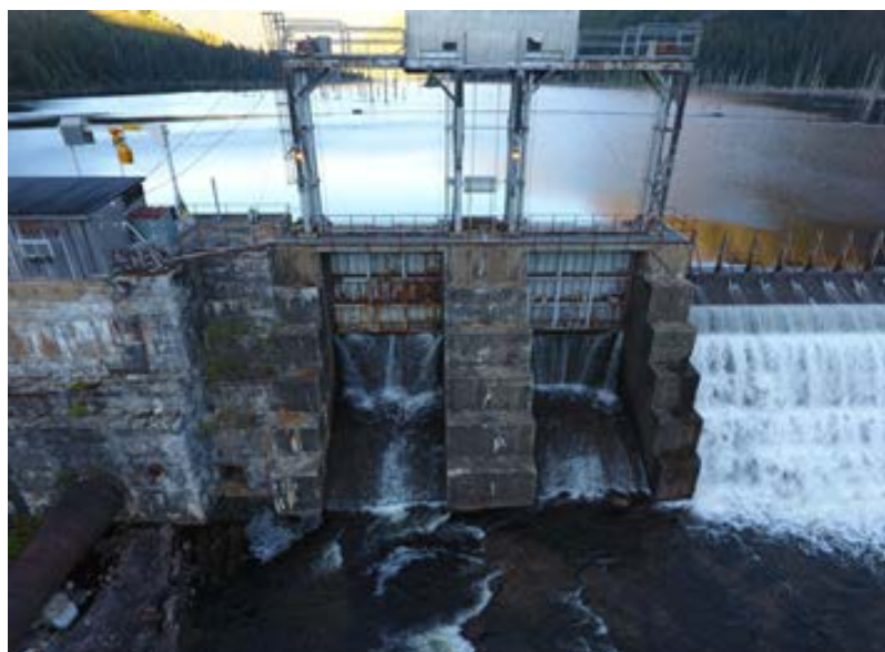
The gated sluiceway at Falls River.
