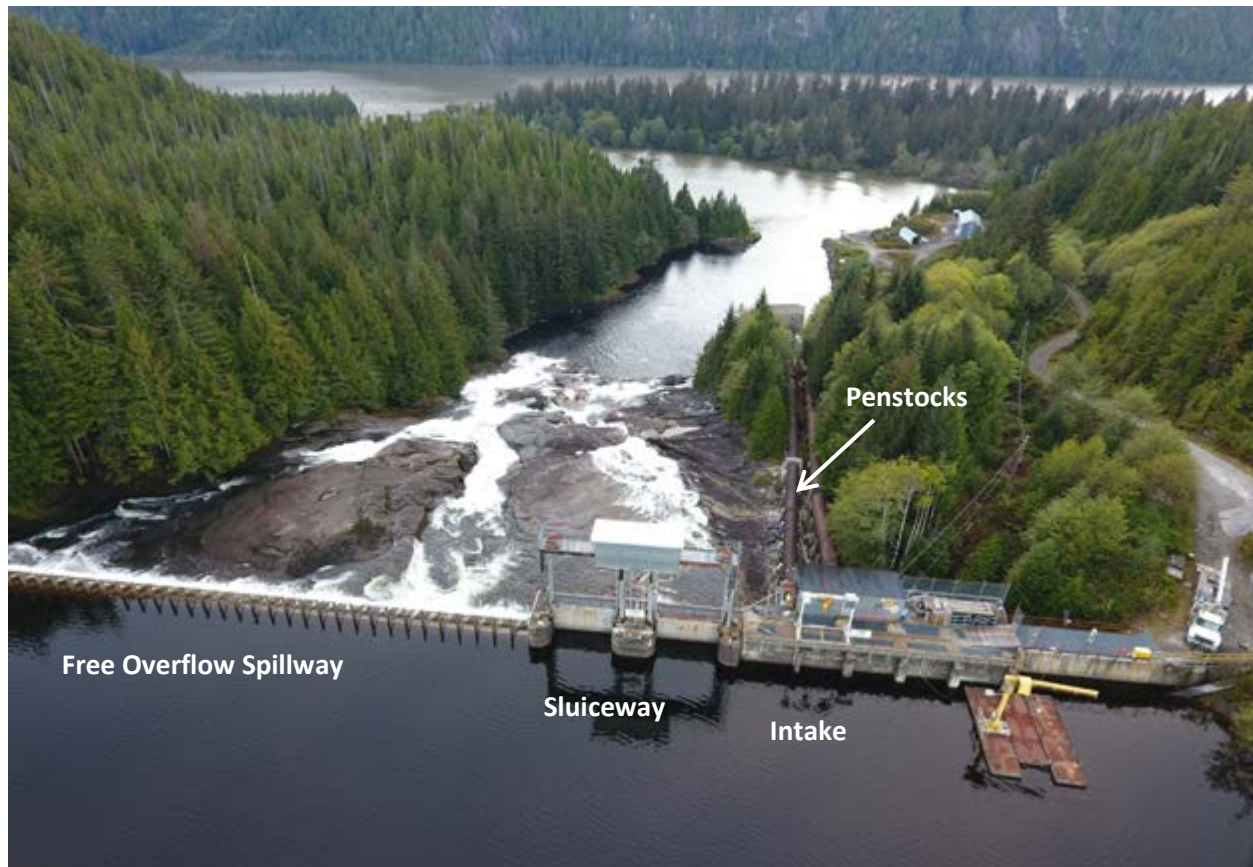
Falls River Dam looking downstream
