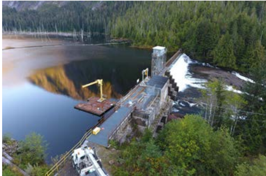
Falls River Dam looking across towards the left abutment
