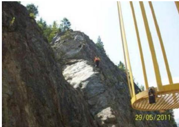
Rock Scaling Activities
