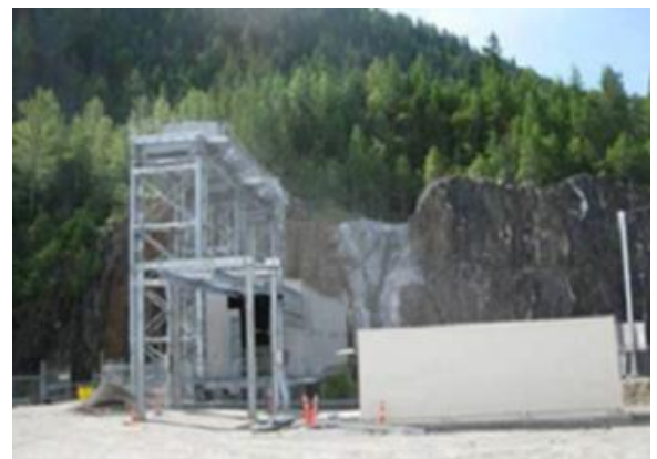
Looking East – Spillway and UPS Building
