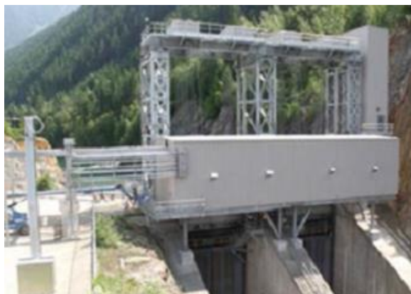
Looking North – Spillway and Hoist House
