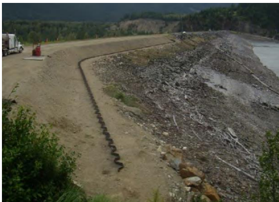
Completed Sheet Pile Wall
