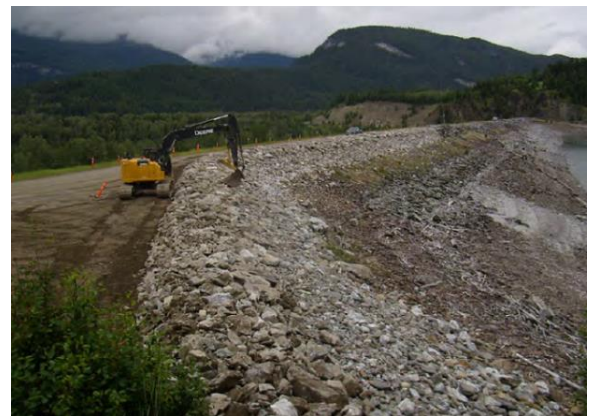
Completed Riprap Slope
