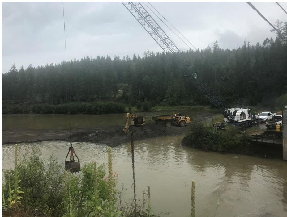
Figure 6 Wilsey Dam headpond silt dredging (August 2019).
