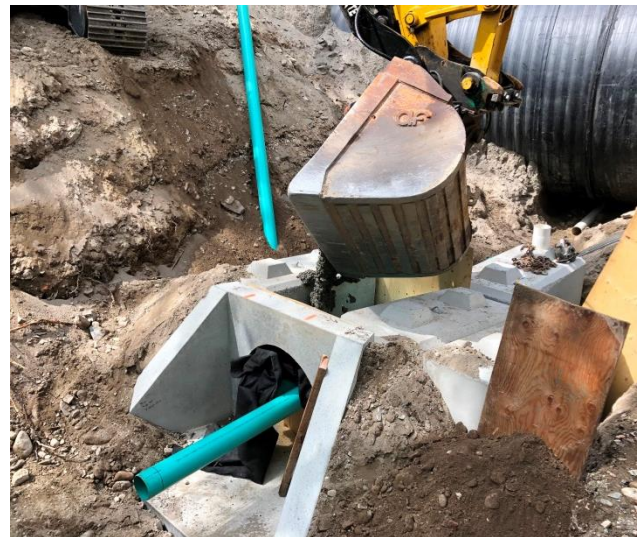
Figure 5 Repairing a damaged weld inside the penstock (left) and installation of a weir to monitor potential leakage at a penstock elbow (right).
