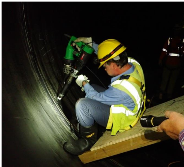
Figure 5 Repairing a damaged weld inside the penstock (left) and installation of a weir to monitor potential leakage at a penstock elbow (right).
