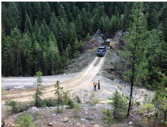
Figure 7 (Left) On commencement of dam crest removal. (Right) On completion.
