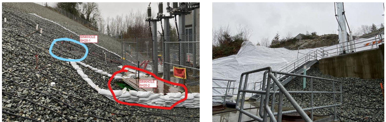
Figure 4 Ruskin Dam left abutment as at 8 January 2021.
