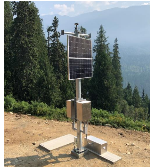
Figure 16 A new continuous Global Positioning System tower on Downie Slide.
