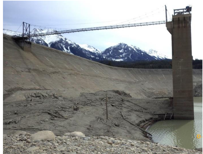
Figure 14 La Joie Dam and intake tower at low reservoir.
