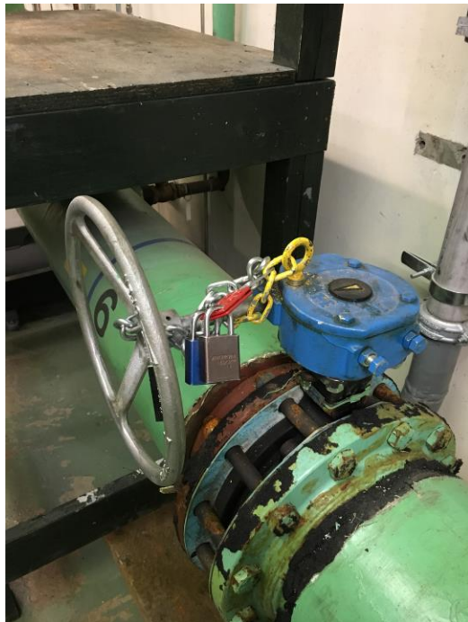
Figure 10. PSSP tag, WPP and system locks
