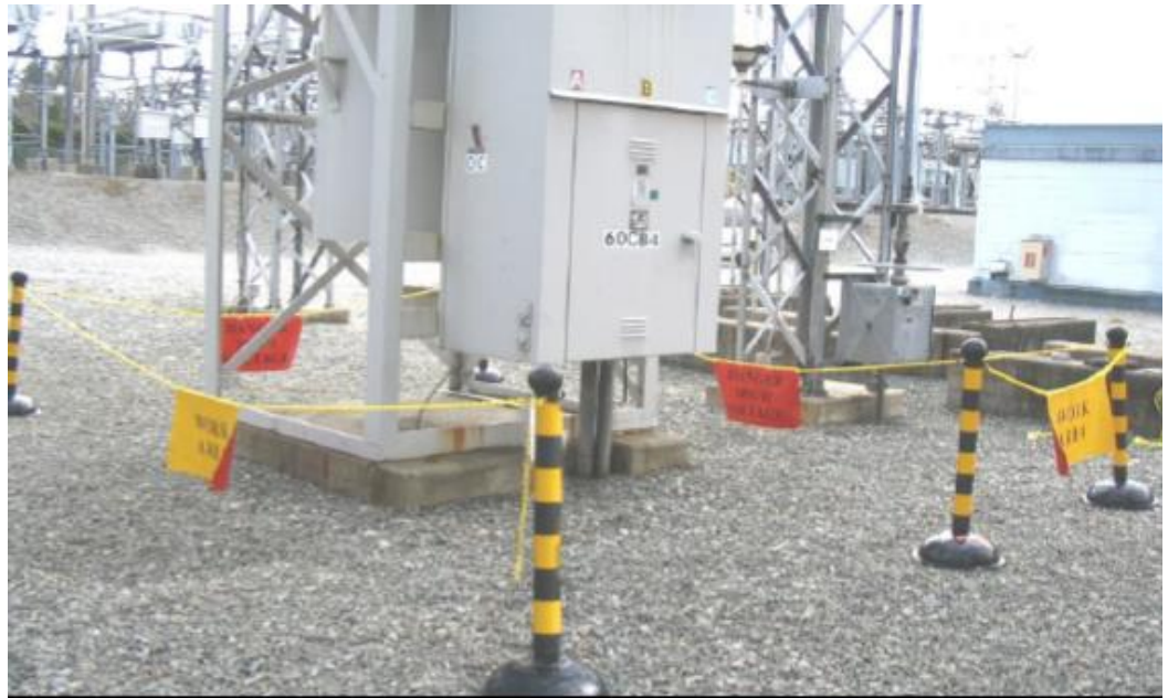
Figure 3. Work area barriers defining safe work area
