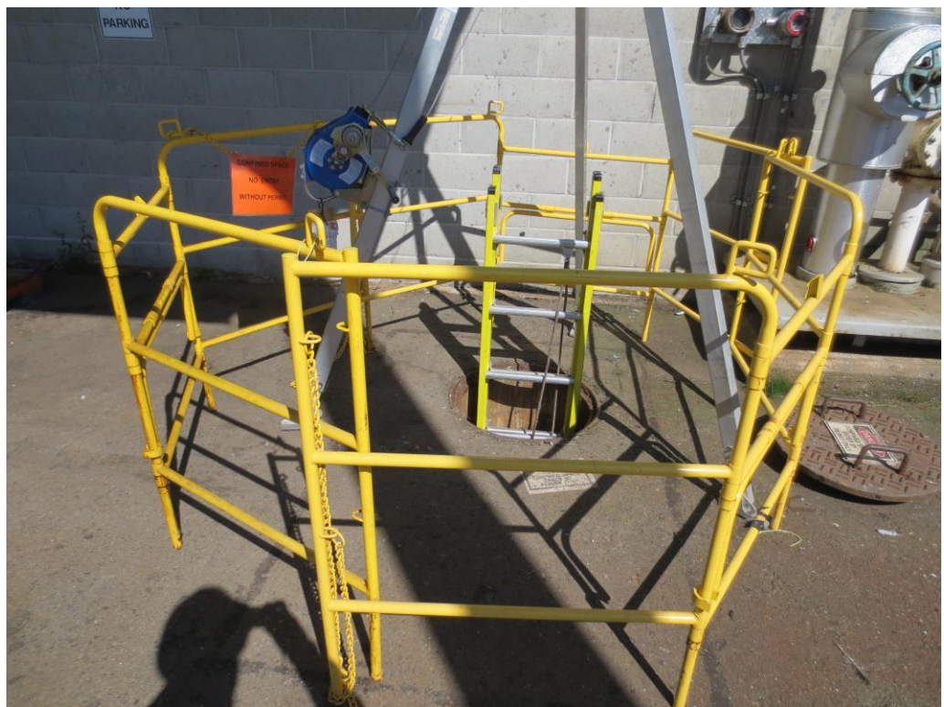
Figure 4. Work area barriers defining a hazard zone
