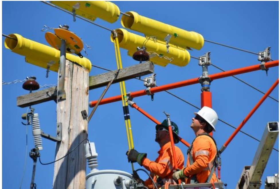
Figure 5. Use of live-line tools
