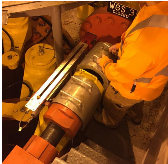
Figure 9. Worker applying mechanical blocking (horseshoe) to a hydraulic cylinder
