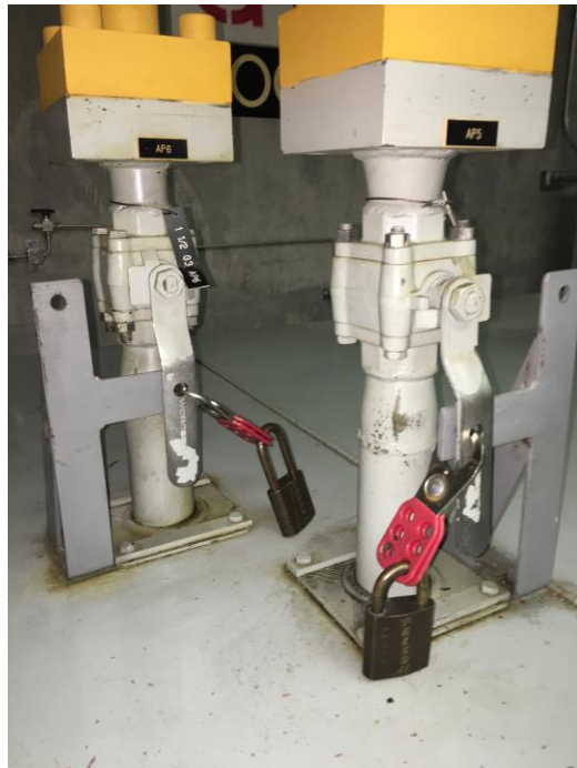
Figure 10. PSSP tag, WPP and system locks
