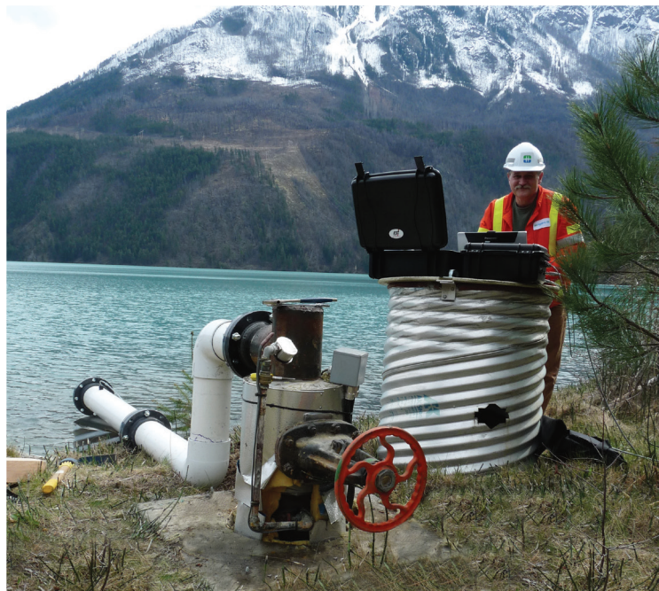
Relief well upgrade at Bridge River
