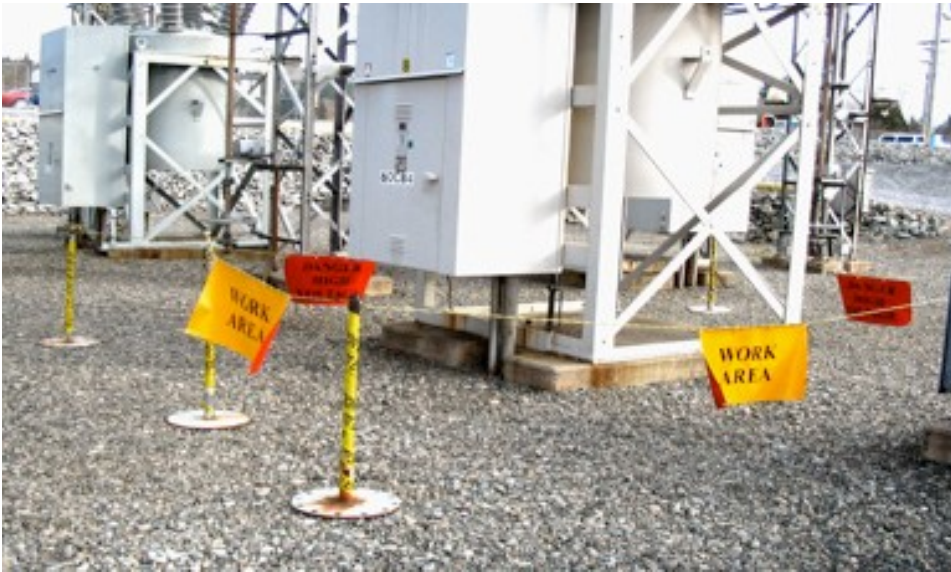
Rope barrier using on-site fabricated steel stanchions
