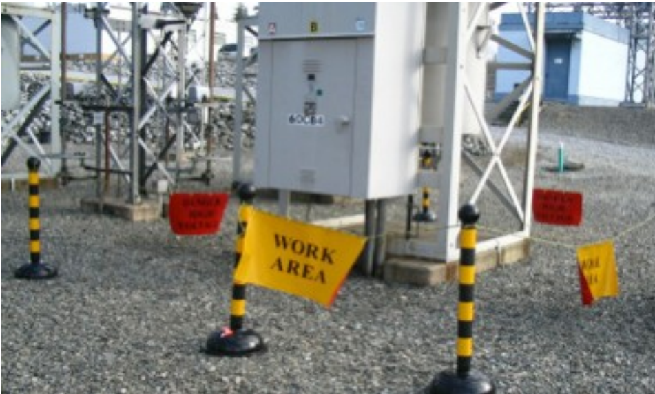
Rope barrier using Bradylink stanchions stock # 92112. Barrier bases weighted with sand or water.
