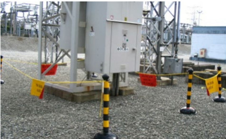
Bradylink plastic chain and barrier stanchions. Barrier bases weighted with sand or water.
