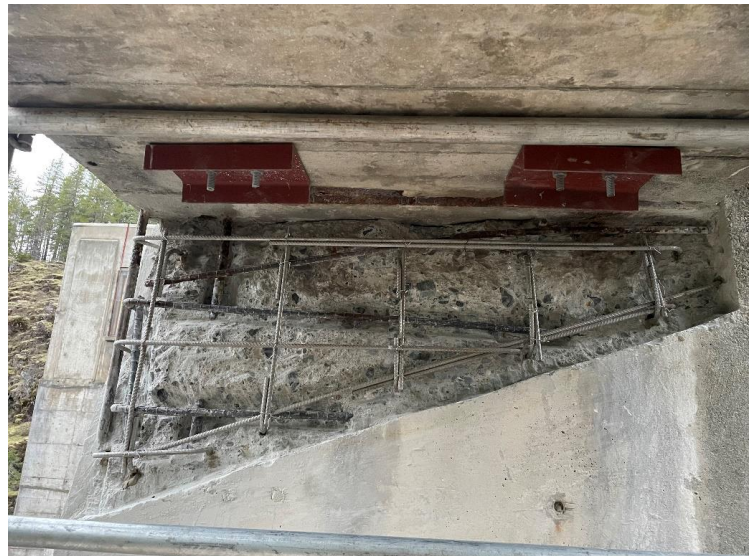
Figure 4 Ladore spillway walkway bridge concrete repair.
