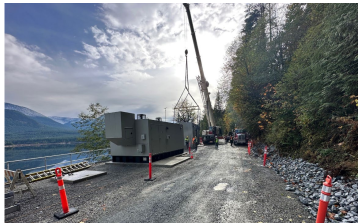
Figure 8 Coquitlam-Buntzen Tunnel Inlet refurbishment. Left: new concrete pier nose between the two intake operating gates. Right: power and control buildings being installed; slope stability upgrade in foreground.
