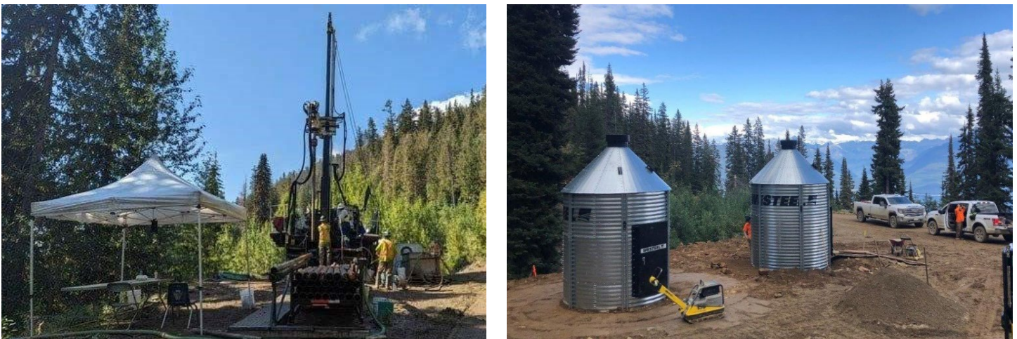
Figure 10 Drilling (left) and installed instrumentation shacks (right) at Little Chief Slide.
