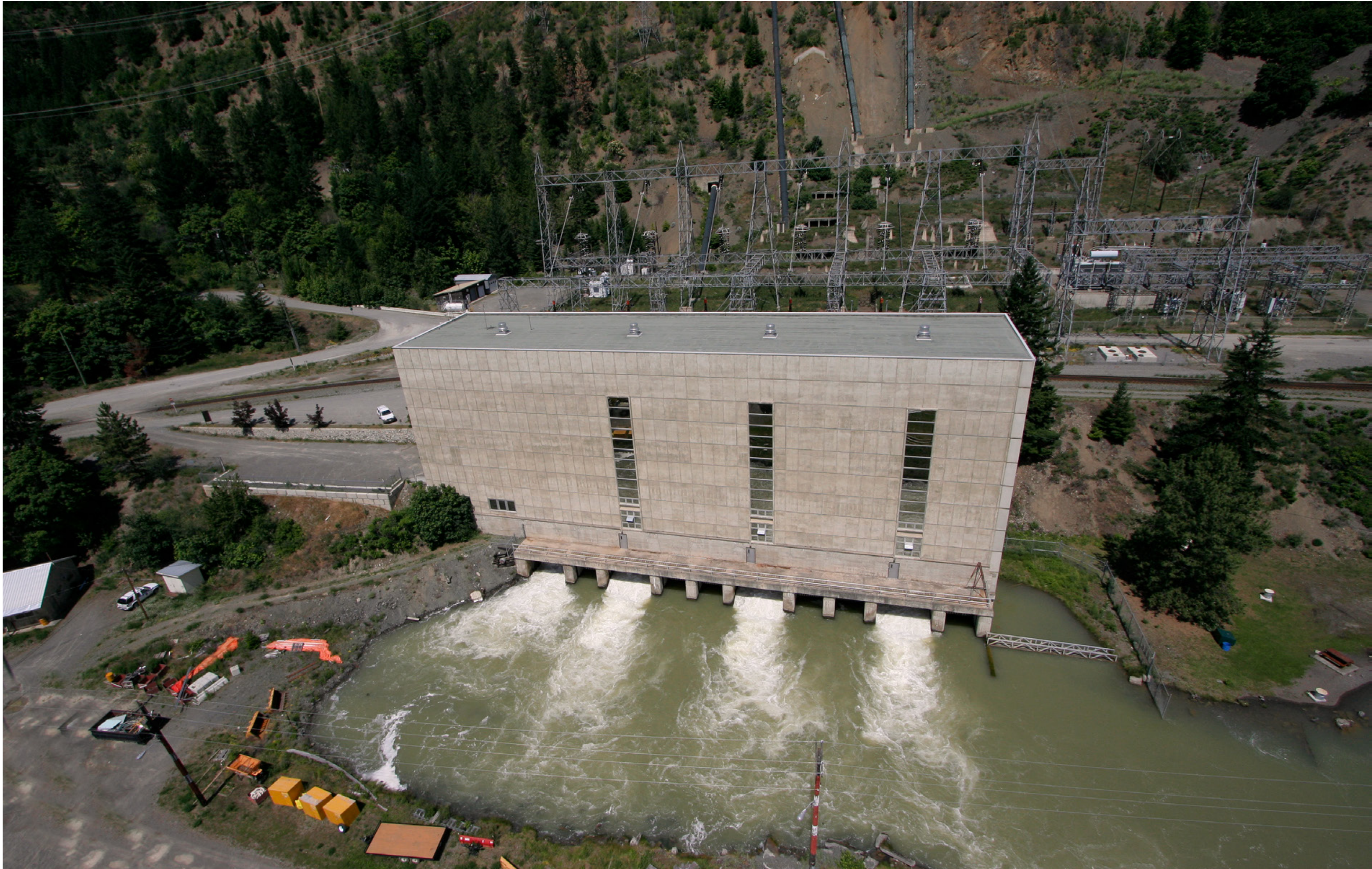
Aerial view of Bridge River Generating Station—Unit 1
