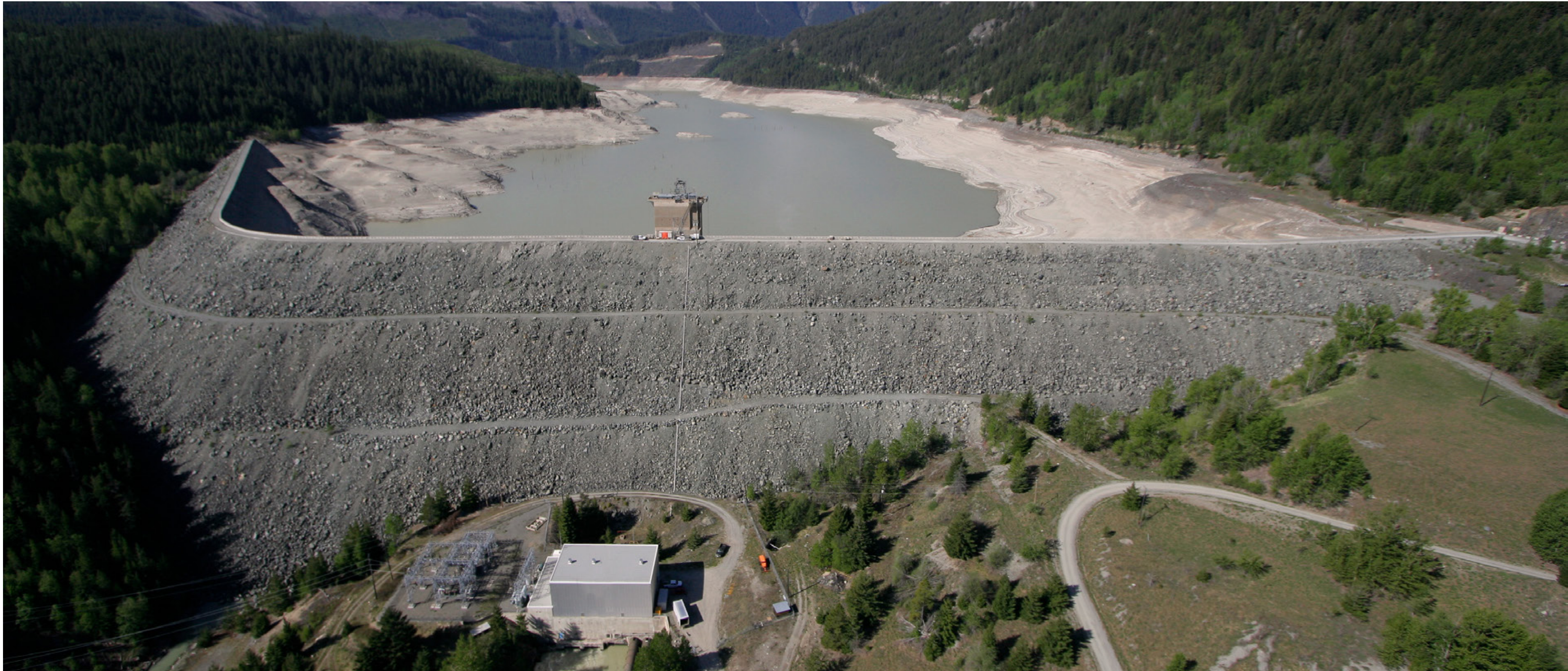
LaJoie Dam with Downton Reservoir in the background and a 25 MW powerhouse in the foreground
