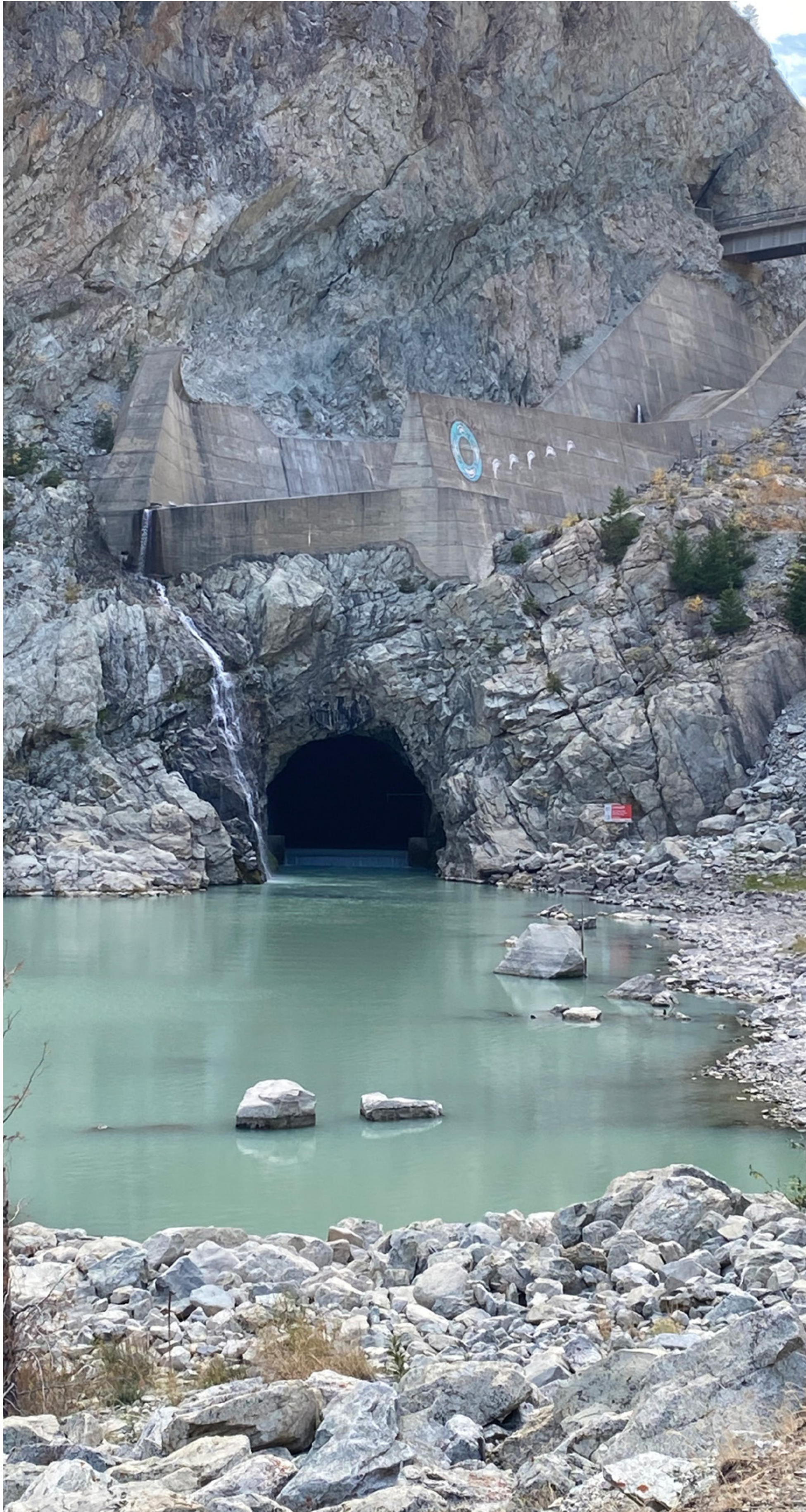
Terzaghi spillway and low level discharge outlet
