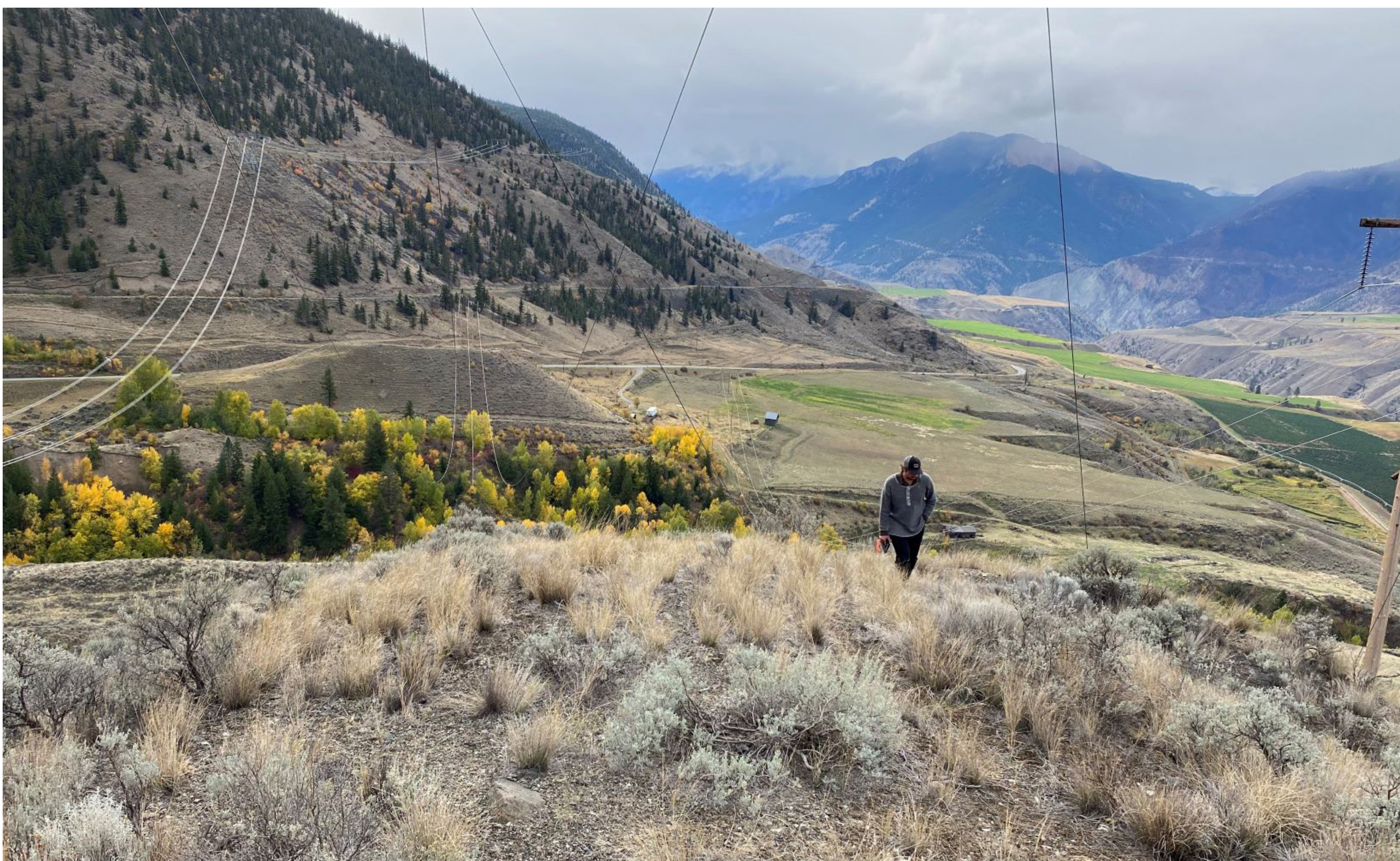
Field work for the Bridge River Transmission Project
