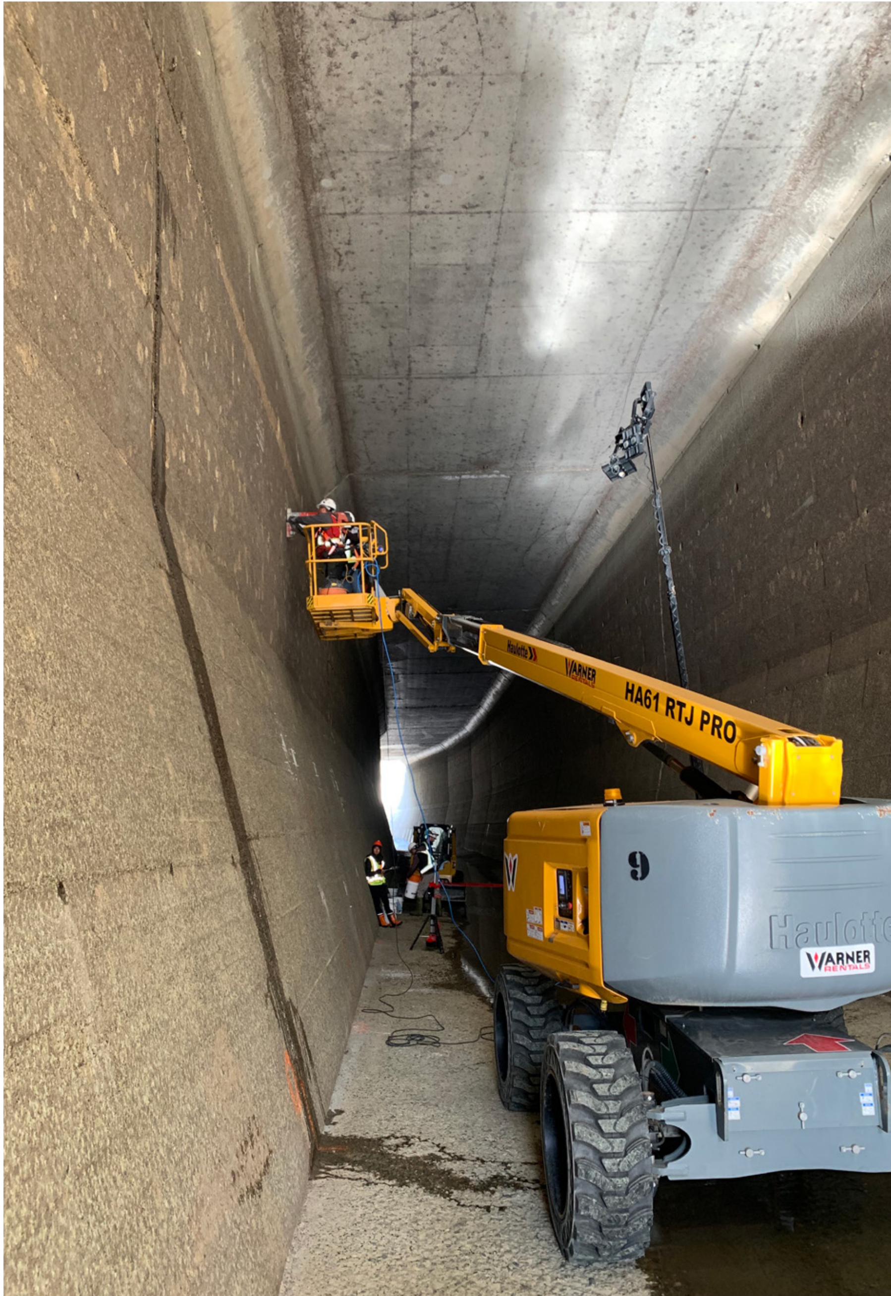
Crews extracting coring samples in Seton Canal, spring 2022
