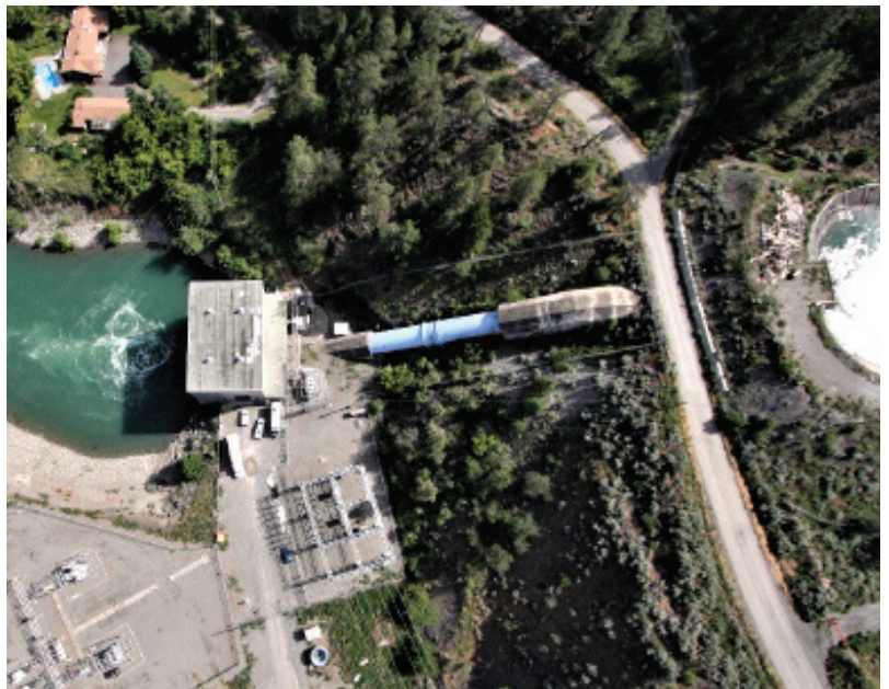
Seton Generating Station
