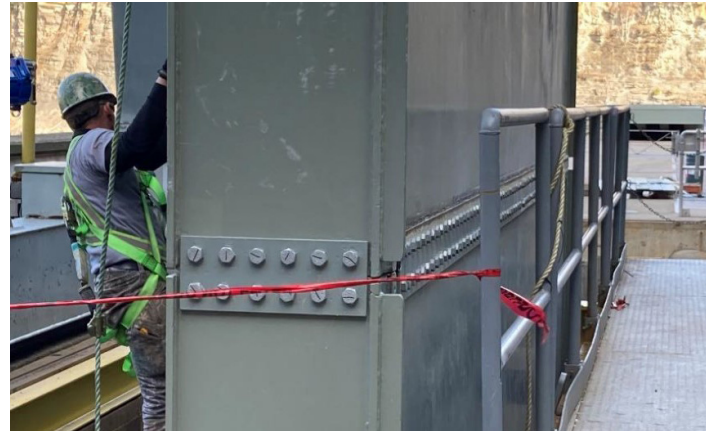
Refurbished PCN draft tube maintenance gate section.
