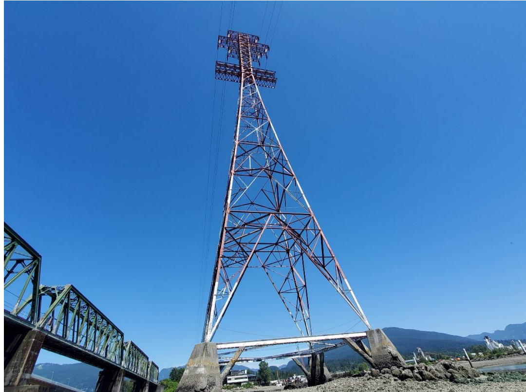
Structure 689 facing North (taken during the low tide)
