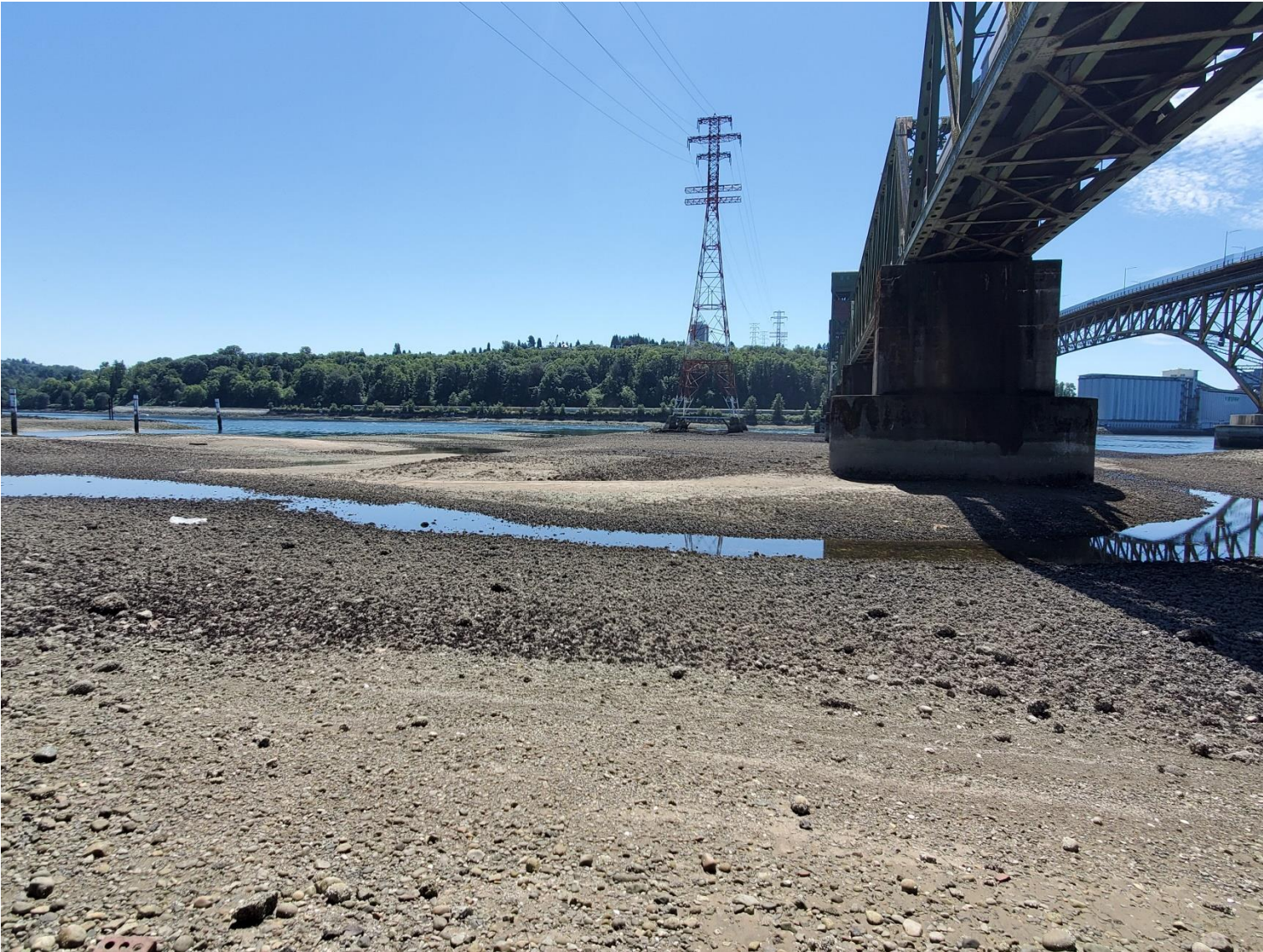
Structure 689 facing south (taken during the low tide)
