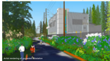
Artist rendering of upgraded substation
