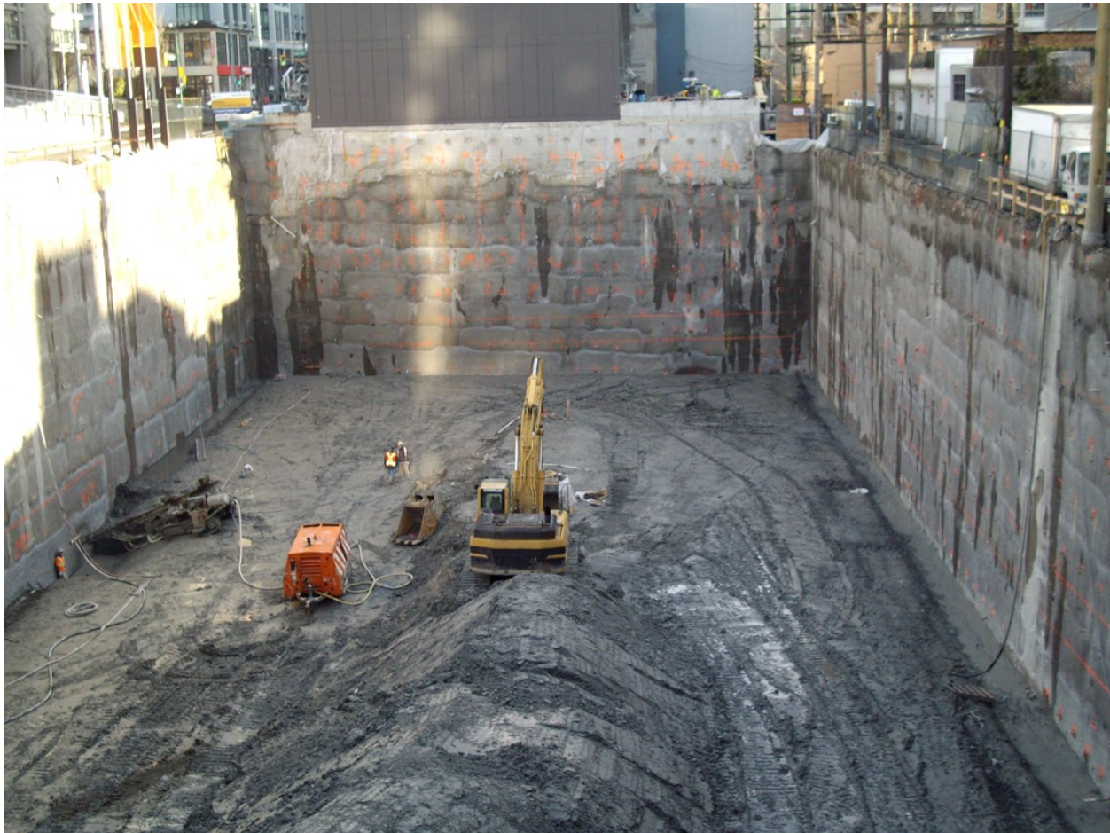
Photo 2-1 Shotcrete and Tie-Back Anchor Retention System—Downtown Vancouver
