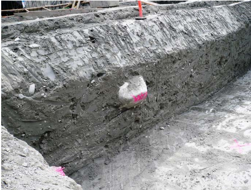
Photo 2-2 Boulder encountered in local downtown Vancouver project
