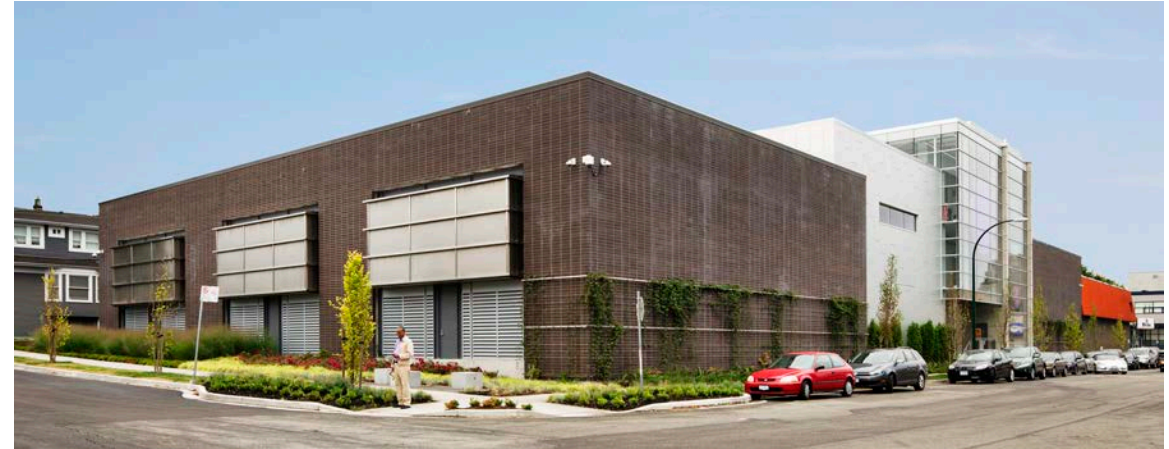
Mount Pleasant substation
