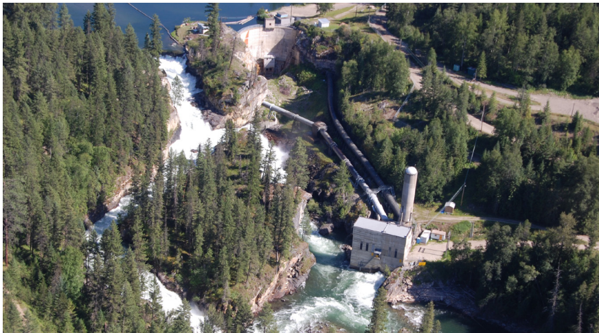
Wilsey Dam and generating station
